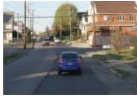
Wide roadway widths on Pittston Avenue without lane edge markings
