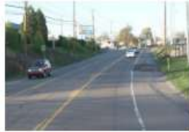
Commercial portion of corridor from transit stop and no sidewalks
