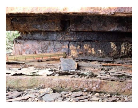
Fracture critical elements & fatigue concerns Constructed in 1914 Weight posting already reduced to 15 tons Inspection required every 6 months AADT: 6,770
