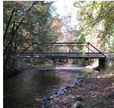
Rehabilitated County Bridge #54706
