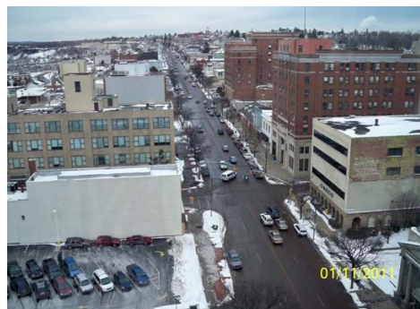
Project View, Looking North on Broad Street
