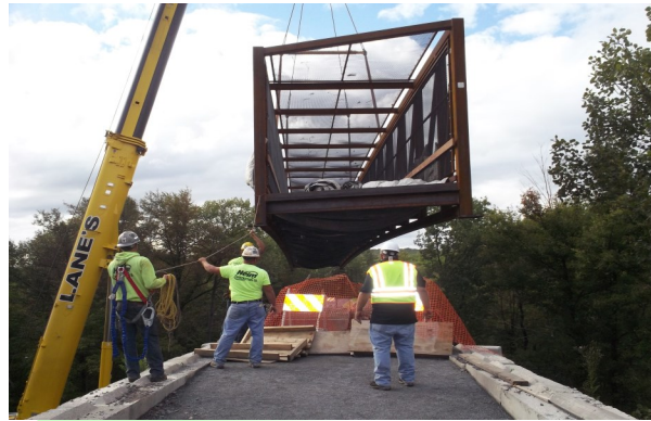
Ashmore Pedestrian Bridge being placed on the GHRT trail.
