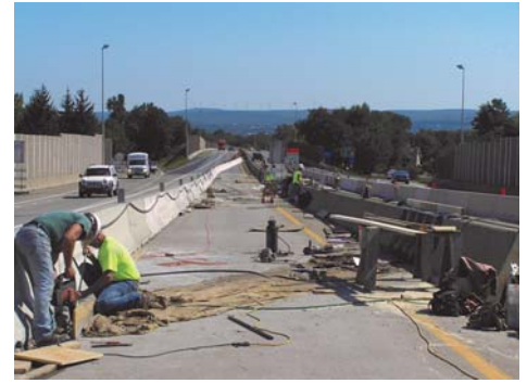
Repair and replacement work continues on the North Crossvalley Expressway
