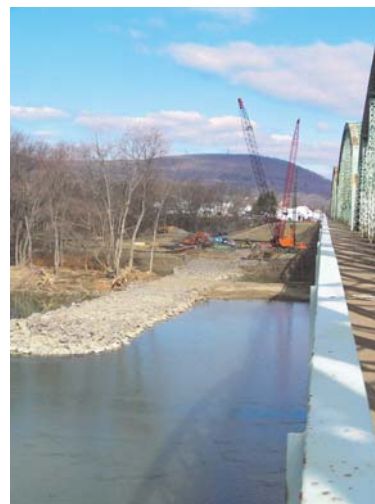
Work continues on the new 8th Street Bridge
