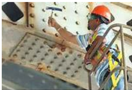
Certified Engineer Performs Inspection of Bridge Substructure
