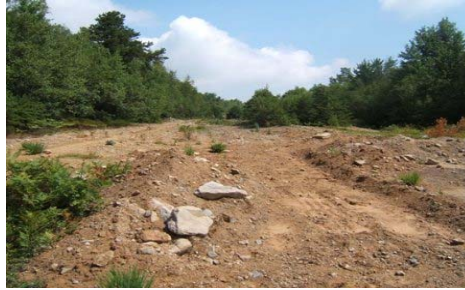
Above: Washed-Out Portion of the GHRT following 2011 Storms. Below: NEG Workers
