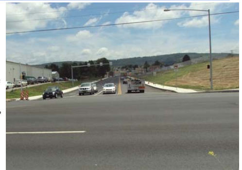
New Coal St. Access Point onto Wilkes-Barre Blvd.
