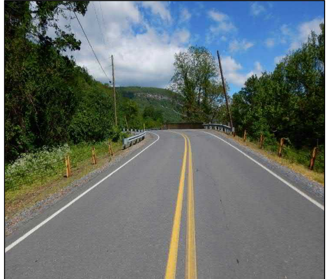
Figure 9 - Looking North along Slateford Road towards Filled-in Slateford Bridge
