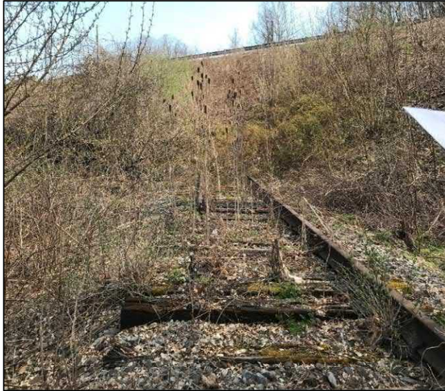
Figure 8 - Looking South at Filled-in Slateford Bridge and track remnants
