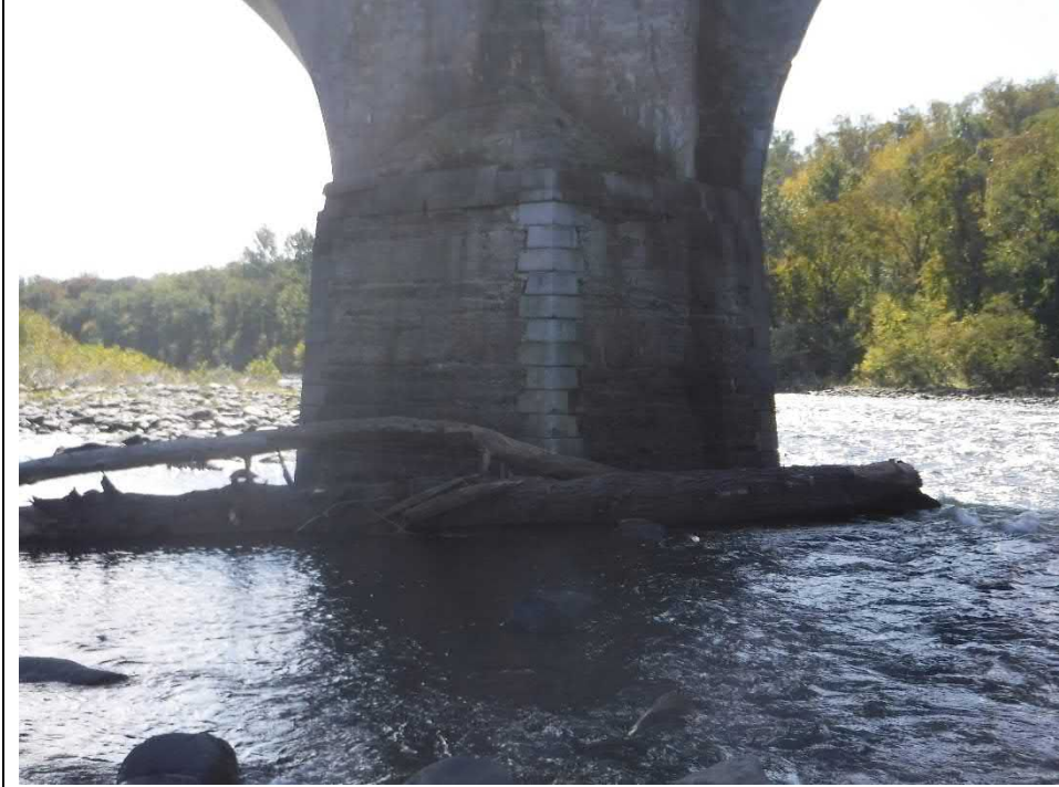
Photograph 13 View of Pier 4 Upstream nose with timber debris
