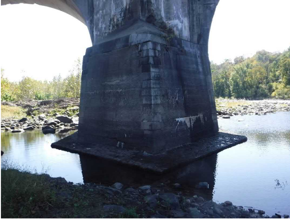
Photograph 19 View of Pier 5 Upstream nose
