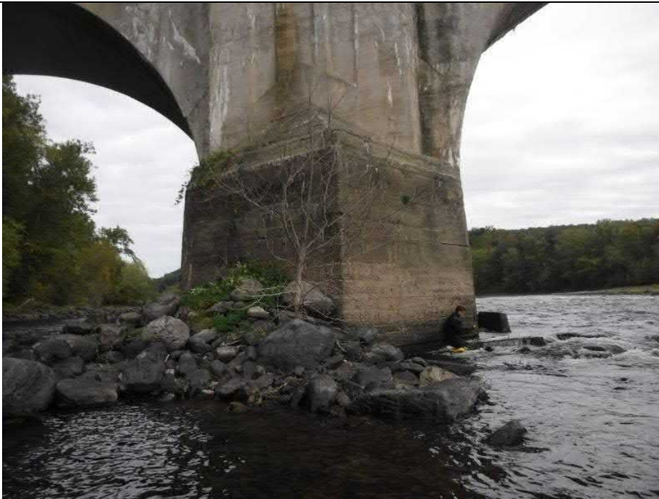
Photograph 8 View of Pier 3 Downstream nose
