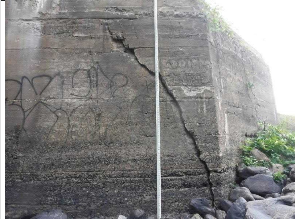
Photograph 11 Structural Crack Pier 3 West elevation. 2" wide full penetration to back side of pier wall downstream
