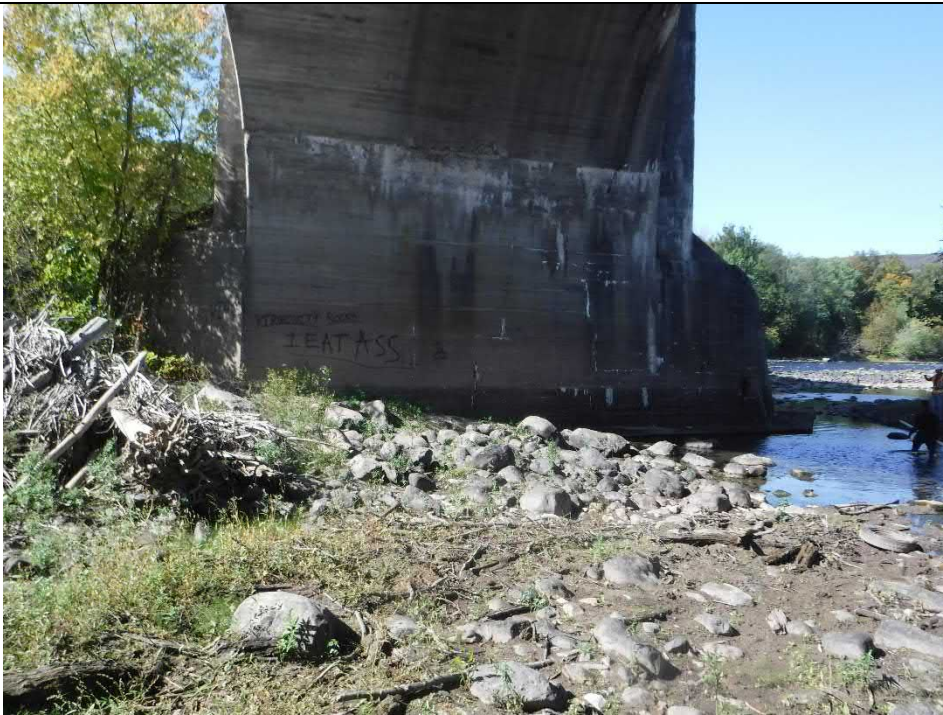
Photograph 20 View of of Pier 5 East Elevation.
