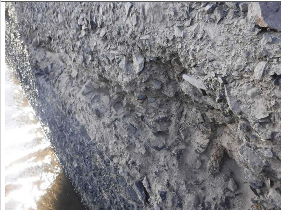
Photograph 12 View of Pier 4, scaling up to 2" penetration above water. Typical of all piers.
