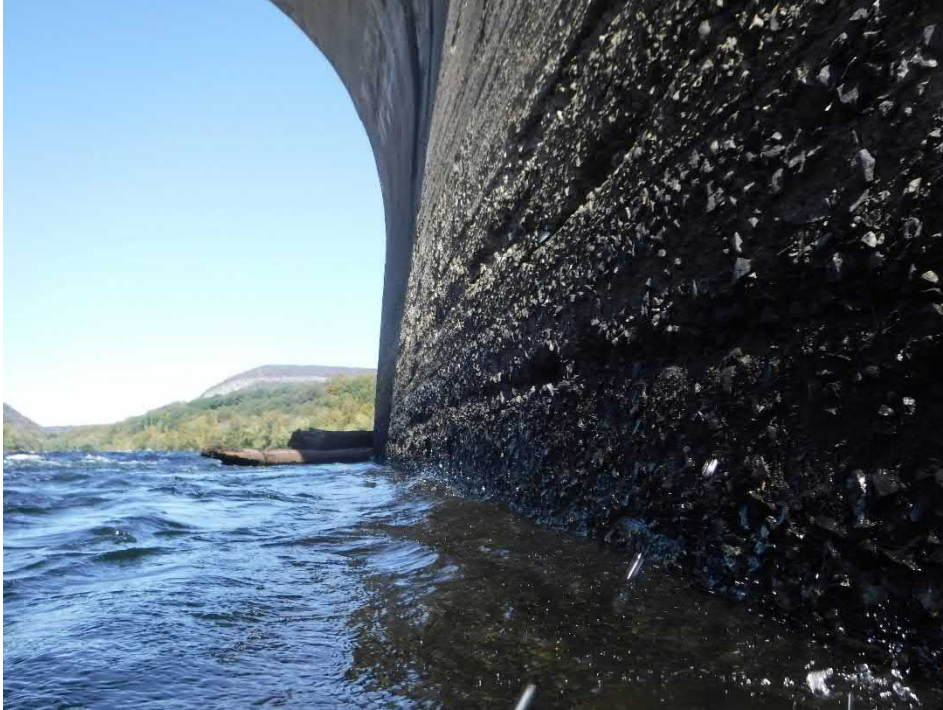
Photograph 15 View of Pier 4 West Elevation.
