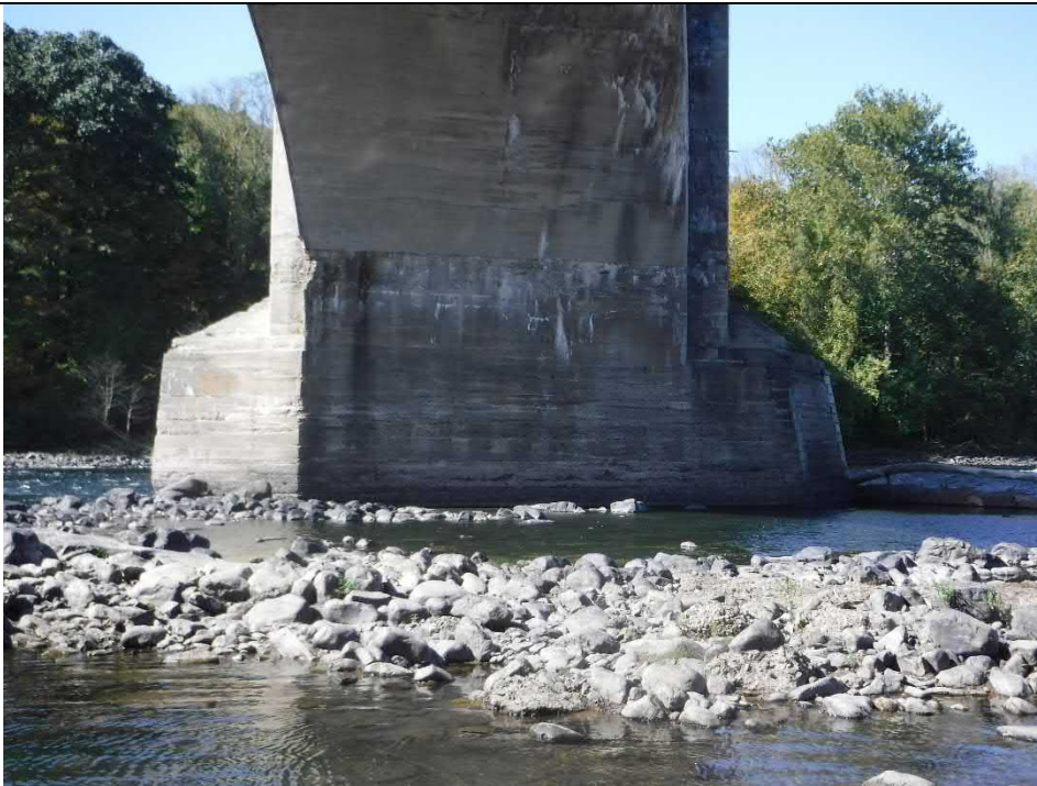
Photograph 16 View of Pier 4 East Elevation.
