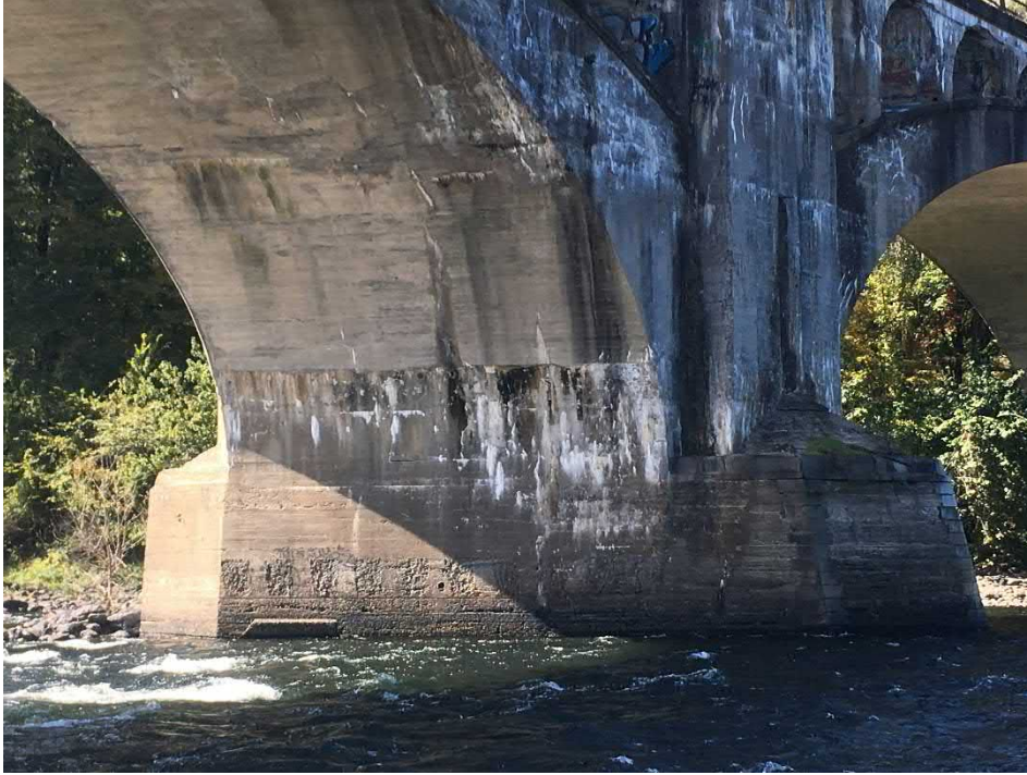
Photograph 7 View of Pier 3 East Elevation
