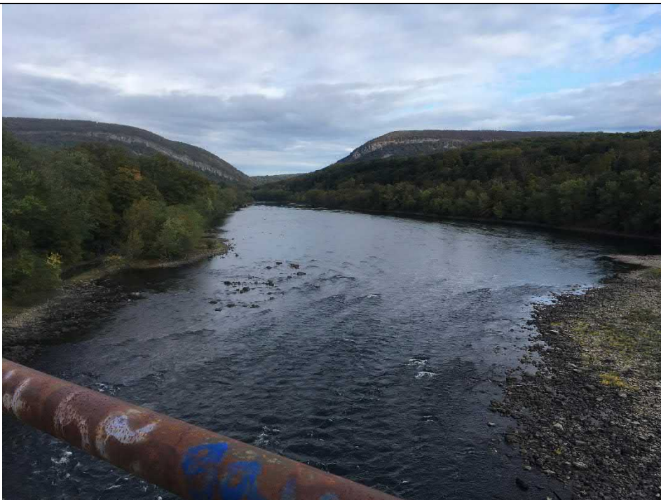
Photograph 4 Overall View of the North / Upstream Channel, Looking North
