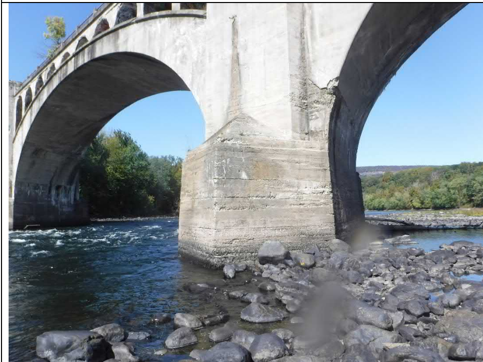
Photograph 14 View of Pier 4 Downstream nose
