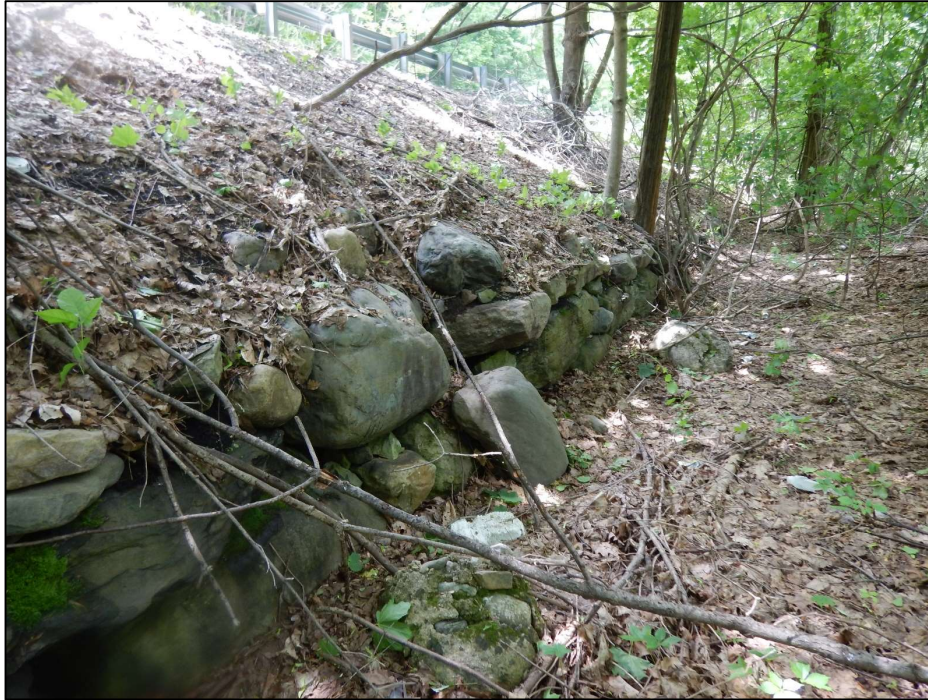
Photo 29 – The typical view of the round stacked stone retaining wall along S.R. 0611 (northernmost section).
