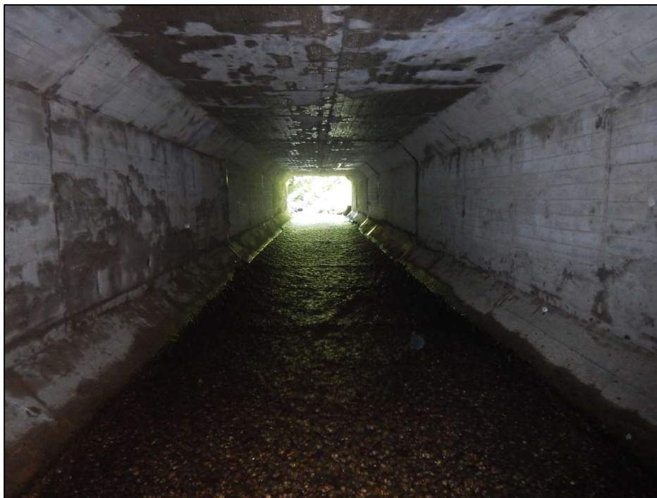
Photo 14 – General upstream view of Span 1 of the PennDOT section from the construction joint looking west.
