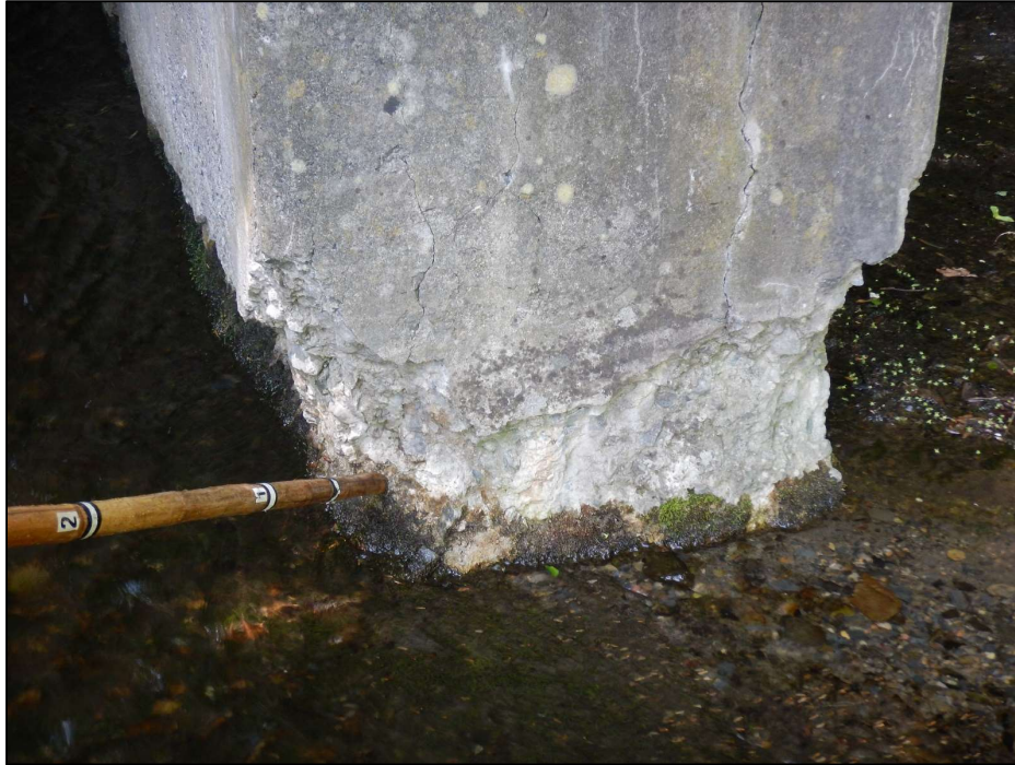
Photo 25 – Abrasion and concrete scaling up to 1'-6" high and 4" deep along the middle culvert wall at the outlet.
