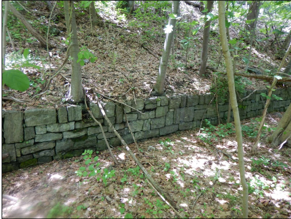
Photo 29 – The typical view of the stacked stone retaining wall along S.R. 0611 (southernmost section).
