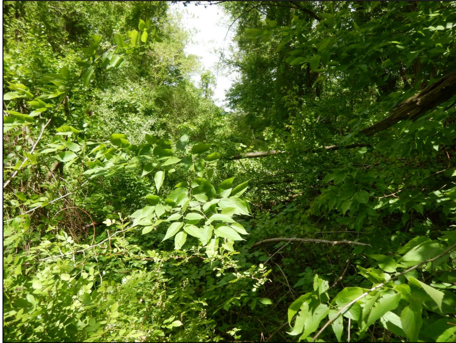
Photo 3 – General view of the PNRRA right-of-way looking north from the culvert. Note the heavy tree and vegetation overgrowth.
