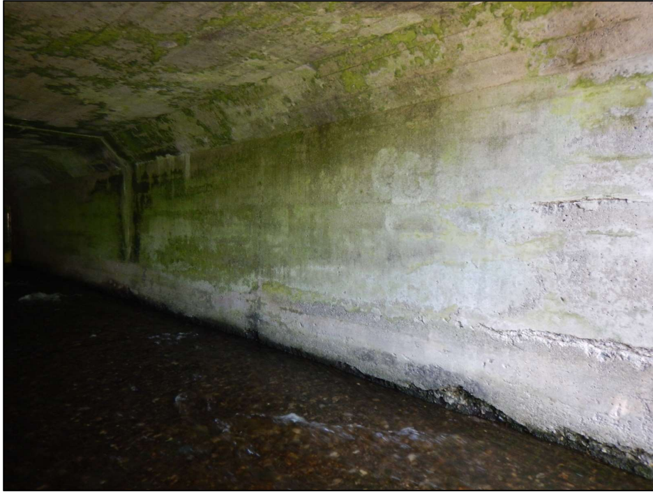
Photo 9 – General view of the south face of the PNRRA middle culvert wall in Span 1 looking northwest from the east facia.
