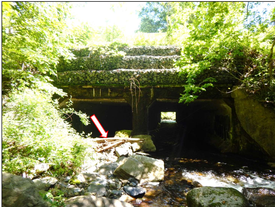
Photo 2 – Left (Upstream) elevation (PennDOT Section). Note the heavily deteriorated fascia with exposed and corroded reinforcement and a gabion basket headwall. Also, note the heavy debris accumulation obstructing Span 2.
