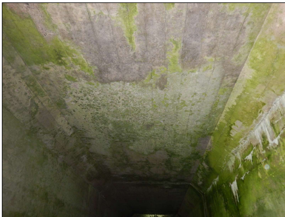
Photo 6 – General underside view of Span 1 from the east fascia of the PNRRA section looking west.
