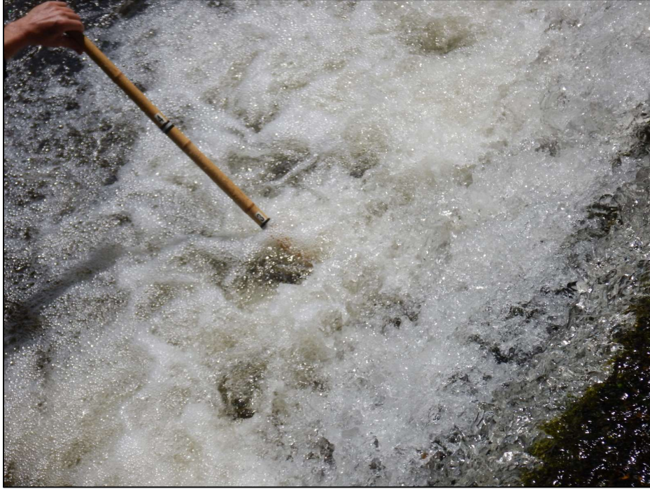
Photo 27 – The outlet apron is undermined up to 1'-0" deep by 1'-0" high in the 3'-0" deep scour hole just downstream.
