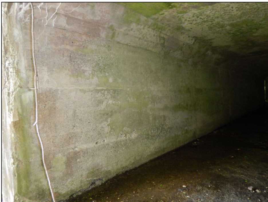
Photo 10 – General view of the north face of the PNRRA middle culvert wall in Span 2 looking southwest from the east facia.
