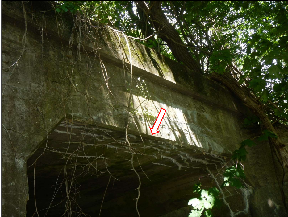
Photo 23 – Close up view of the Span 2 east fascia and headwall. Note the heavy vegetation overgrowth and cracked concrete with efflorescence and stalactites in the top slab.
