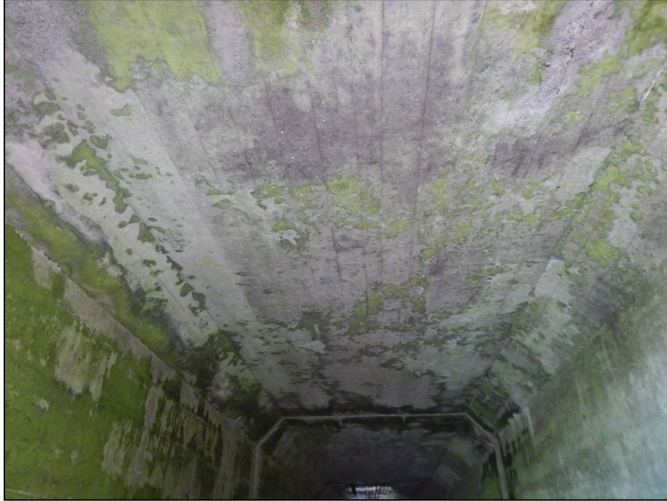
Photo 7 – General underside view of Span 2 from the east fascia of the PNRRA section looking west.
