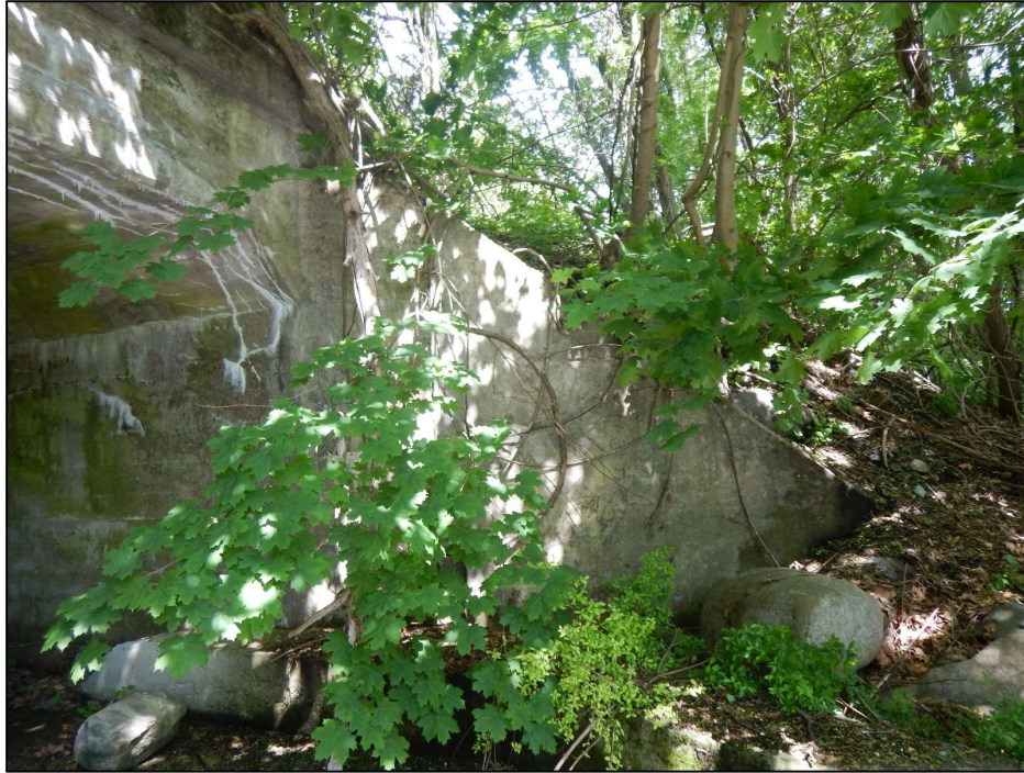
Photo 13 – General view of the northeast wingwall at the outlet looking north. Note the heavy vegetation overgrowth.
