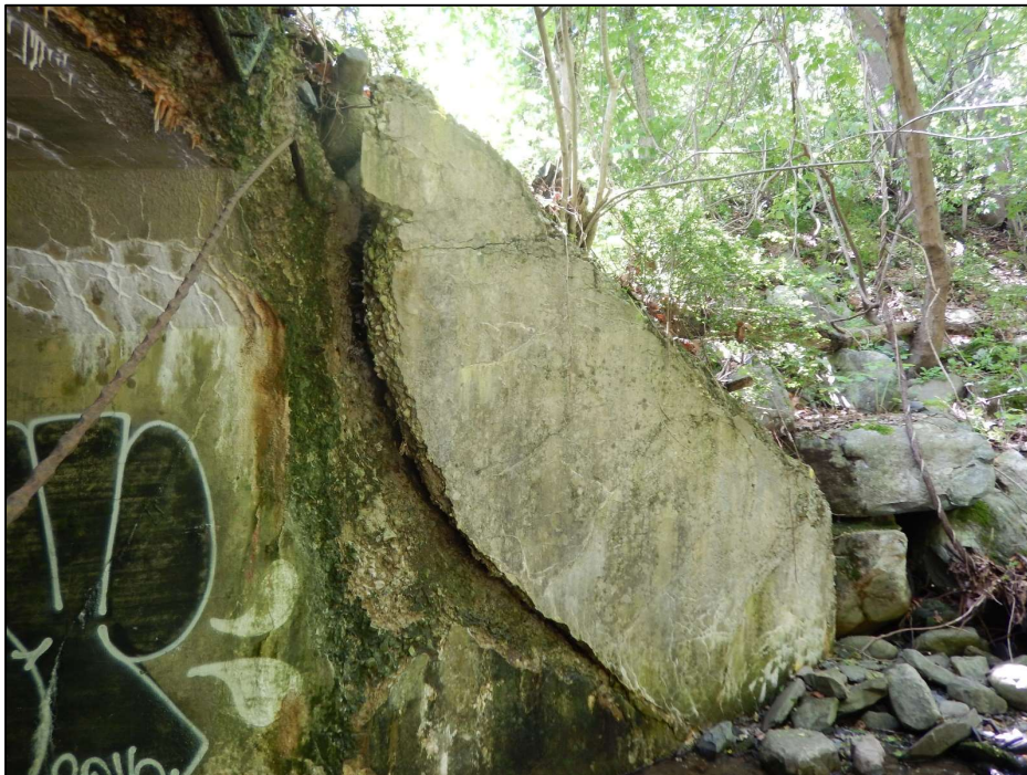
Photo 28 – The southwest wingwall in the PennDOT section (upstream) exhibits severe scale along the interface with the culvert up to 12" deep and leans 7¼" toward the stream.
