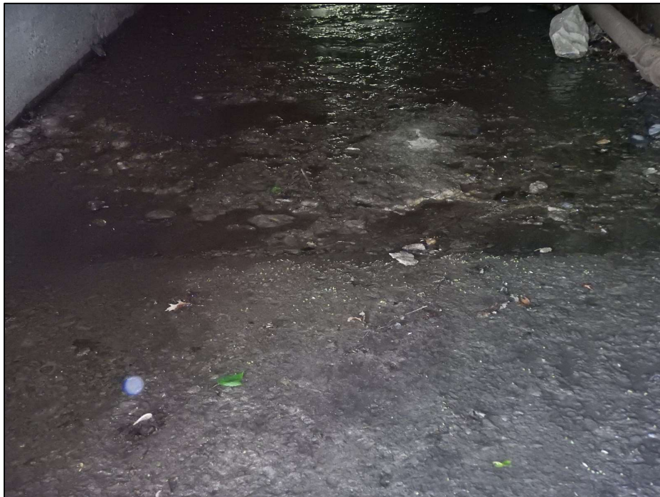
Photo 26 – Heavy abrasion and concrete scaling along the concrete floor. Typical of both spans (Span 2 shown).
