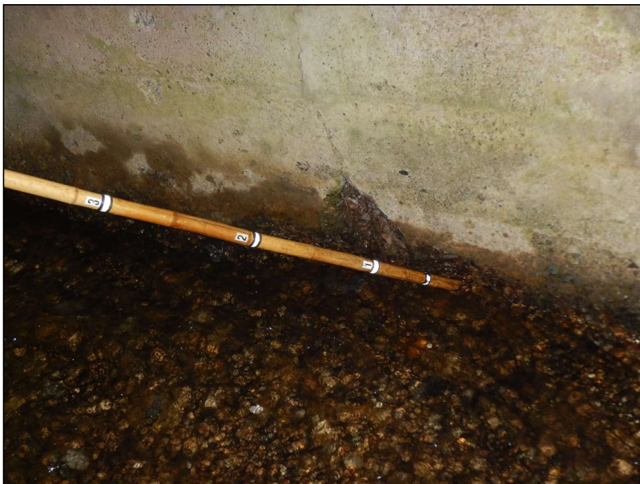
Photo 24 – Abrasion and concrete scaling up to 1'-0" high and 3" deep along the waterline. Typical in both Spans.
