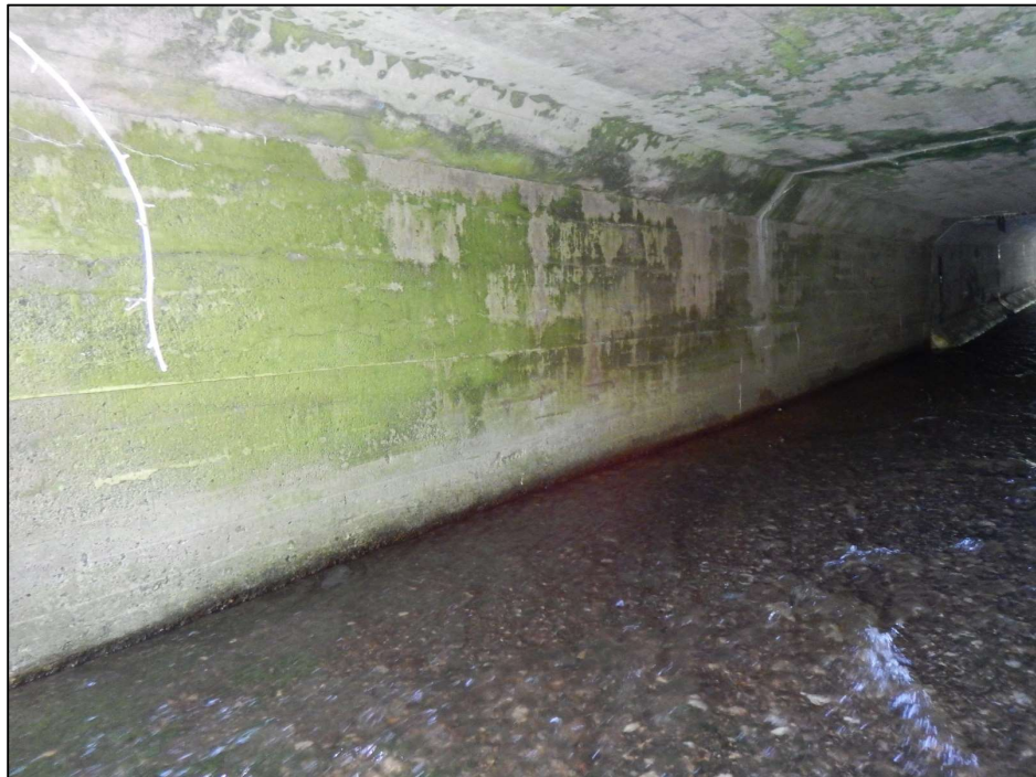
Photo 8 – General view of the PNRRA south culvert wall in Span 1 looking southwest from the east fascia.
