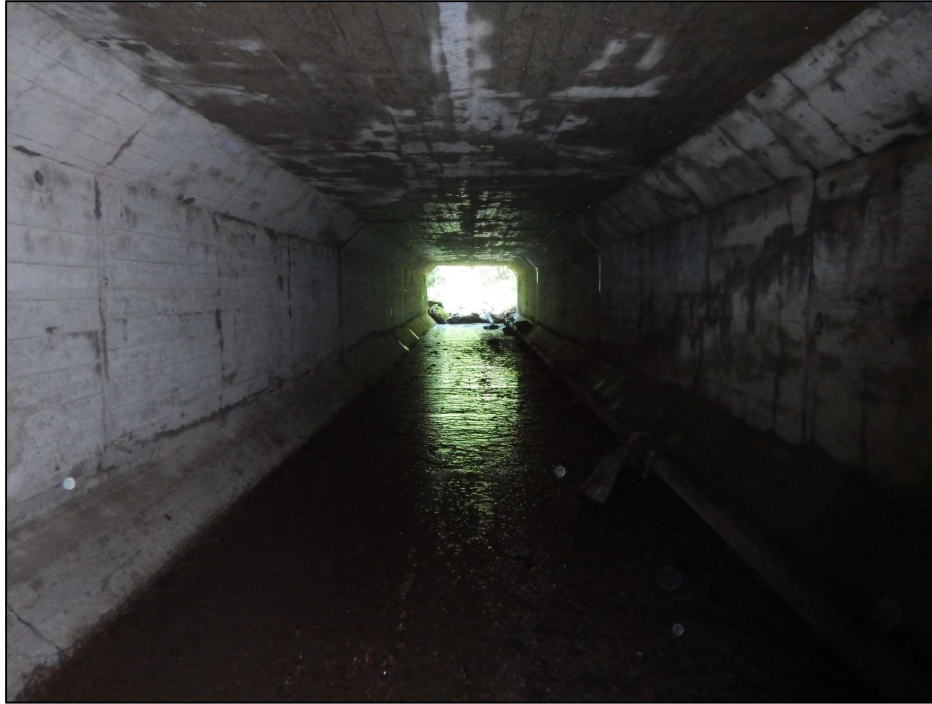
Photo 15 – General upstream view of Span 2 of the PennDOT section from the construction joint looking west.
