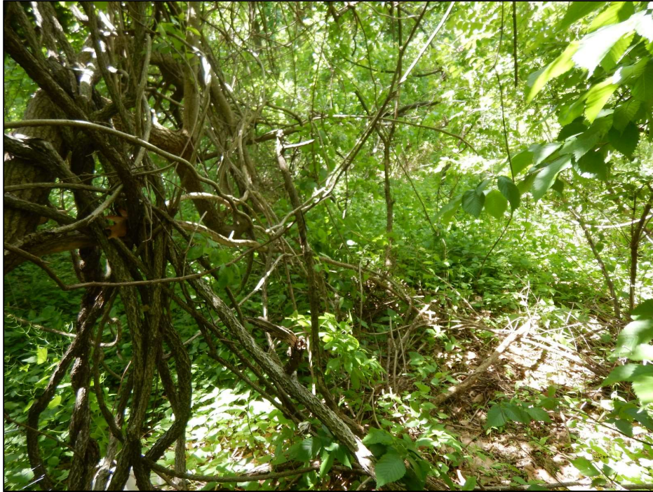
Photo 5 – General view of top side from the northeast corner of the culvert looking southwest. Note the heavy tree and vegetation overgrowth.
