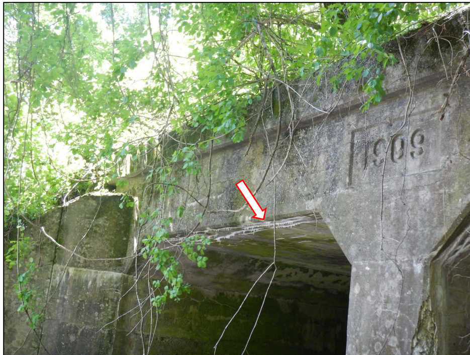
Photo 22 – Close up view of the Span 1 east fascia and headwall. Note the heavy vegetation overgrowth and cracked concrete with efflorescence and stalactites in the top slab.
