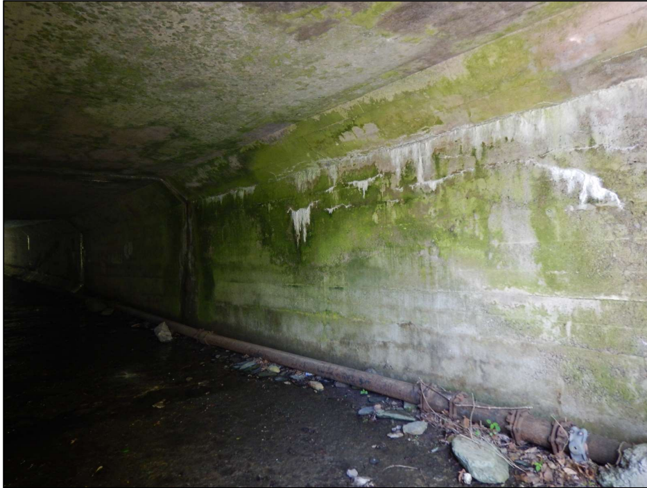
Photo 11 – General view of the PNRRA north culvert wall in Span 2 looking northwest from the east facia.
