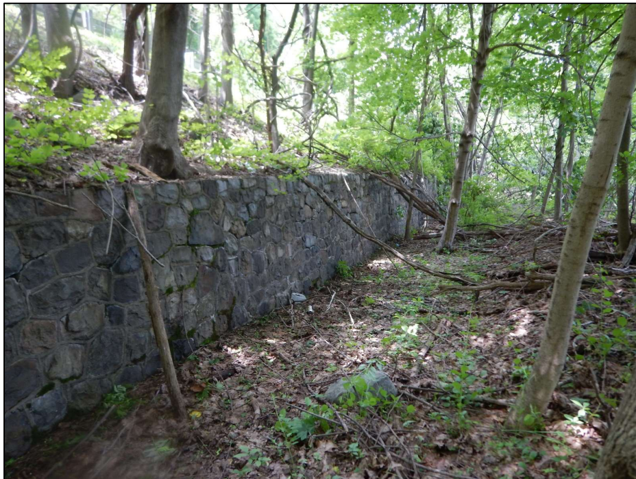
Photo 30 – The typical view of the stone masonry retaining wall along S.R. 0611 (middle section).
