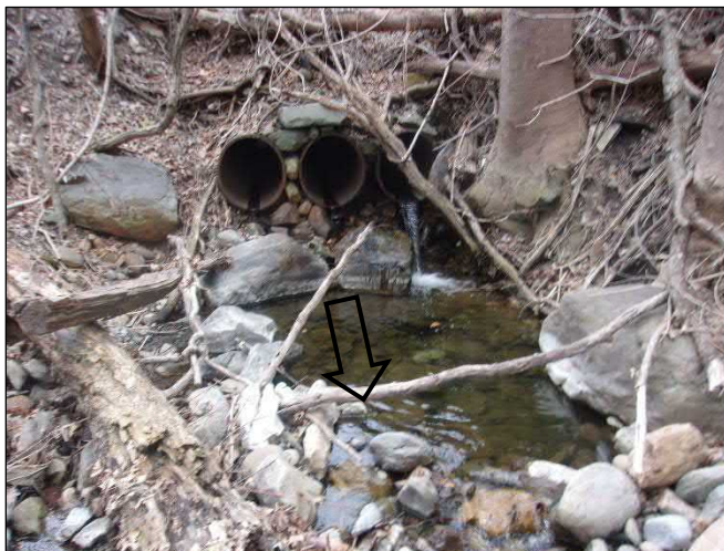
Scour Hole Downstream of Pipes 22, 23, 24
