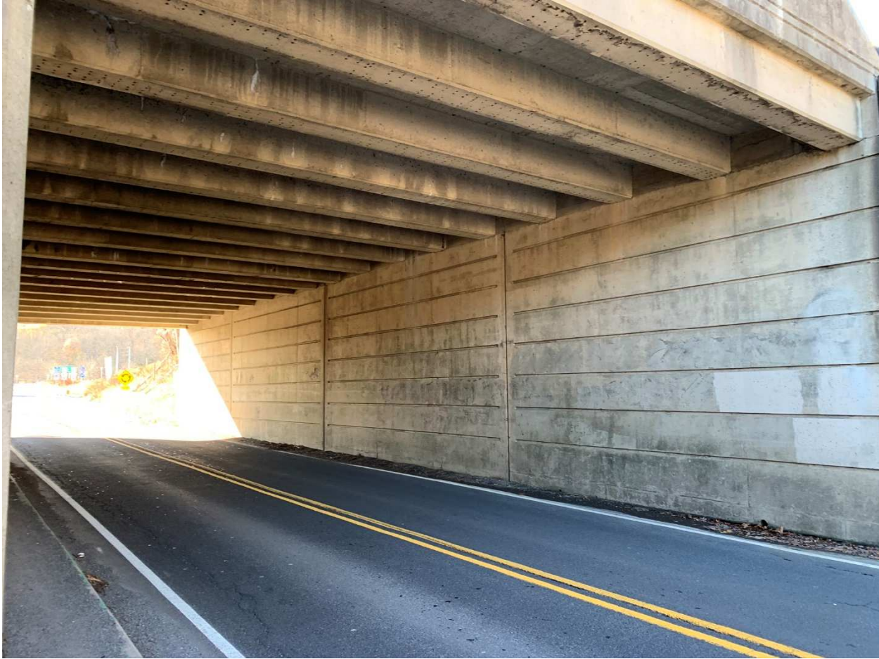
Picture 6: River Road looking Westbound , showing I-80 underpass.
