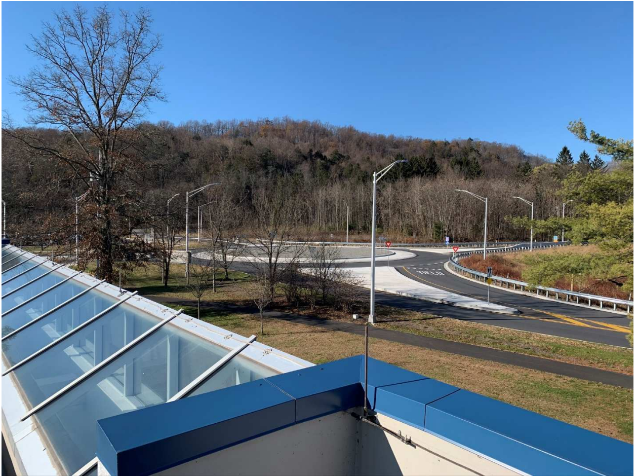
Picture 2: Roundabout intersection at River Road and Broad Street.
