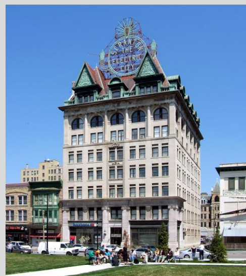
The Scranton Electric Building Built as the Board of Trade Building in 1896 - An example of Beaux Arts style
