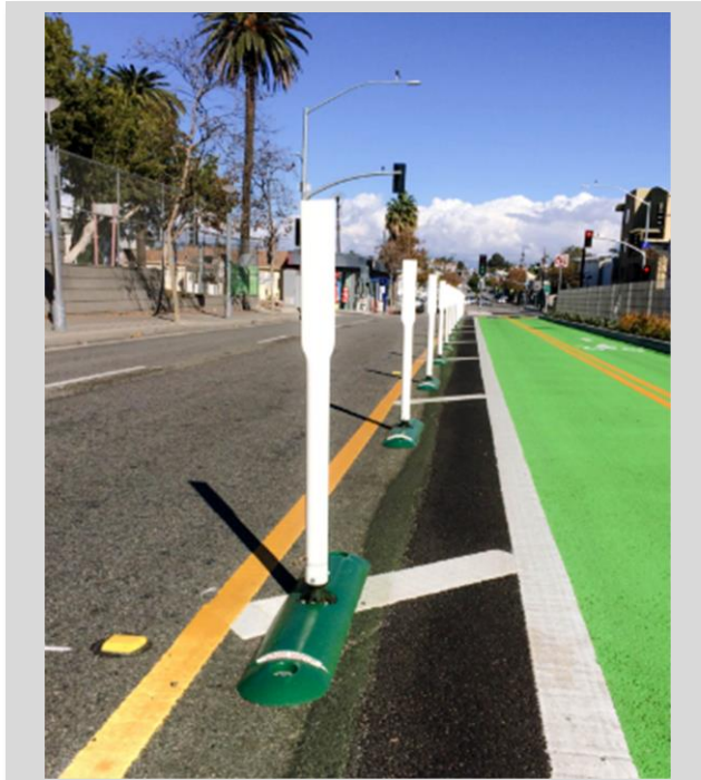
Green-backed bicycle lane pavement markings and plastic delineator posts help to further define a bike lane/cycle track, as well as provide a better sense of security.
