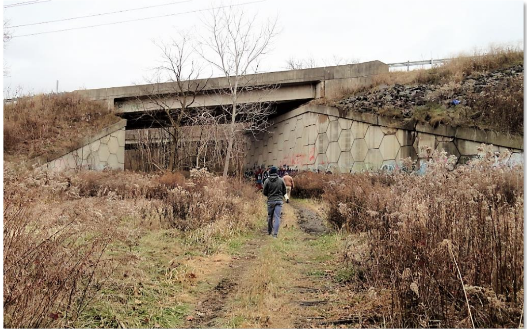
Potential rail-trail at the Route 309 bridges
