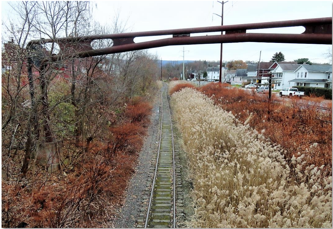
Potential rail-with-trail and historic pipe bridge seen from the Blackman Street Bridge
