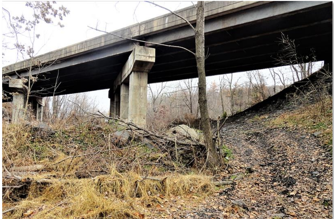
Potential rail-trail at the I-81 northbound bridge
