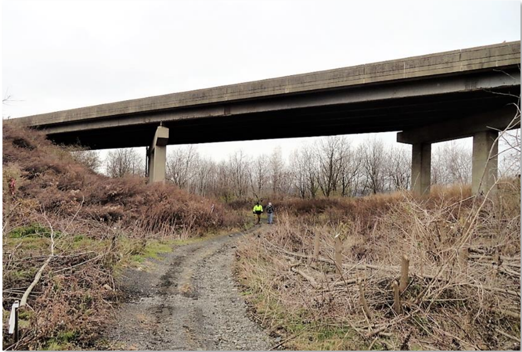
Potential rail-trail at the I-81 southbound bridge
