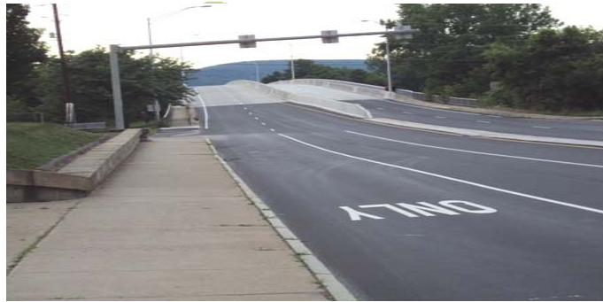
Newly Re-Decked Pierce Street Bridge, Kingston/Wilkes-Barre, opened to traffic in June
