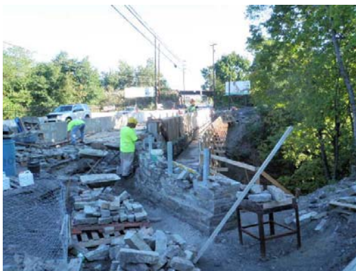
Work continues on the River Road project in Luzerne County.
