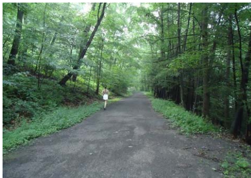
Section of Back Mountain Trail needing rehabilitation
