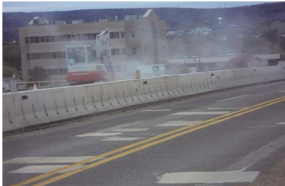
Work Continues on the Pierce St. Bridge Deck Replacement Project
